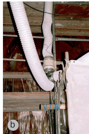
Fig. 3.9.6. Dust and debris produced during laser cleaning are removed by an integrated extraction system. Sigismund's Chapel, Wawel. Photo by J. Marczak.
